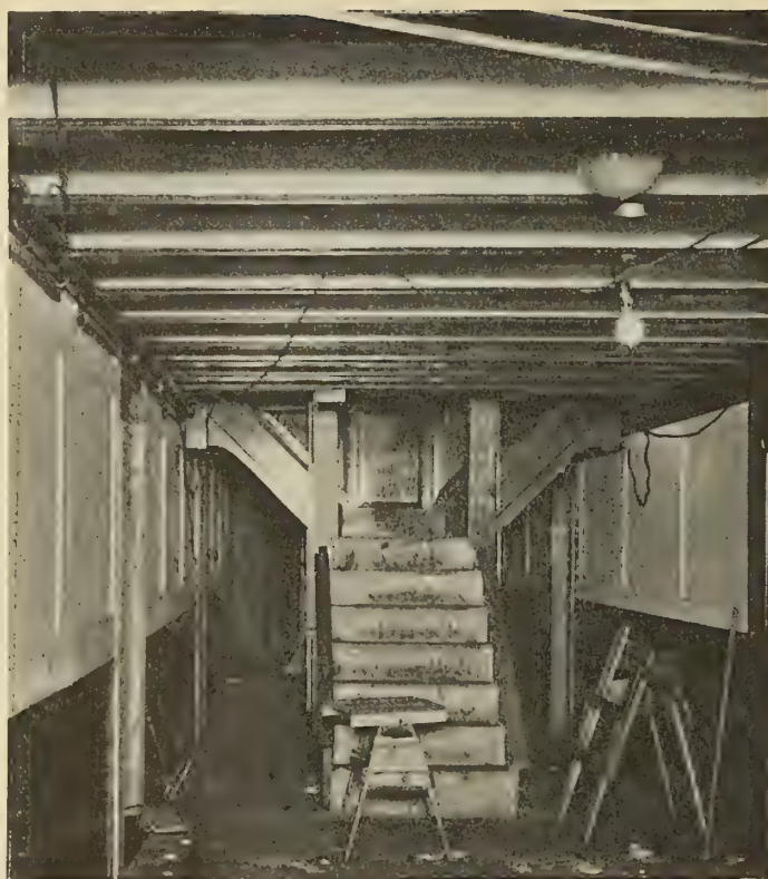
( Photograph by Morse Dry Dock & Repair Company ) Fig. 11.—Stairway and Panel Work in Passageway
